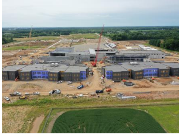
Aerial view of the building looking South (08/12/2022)
