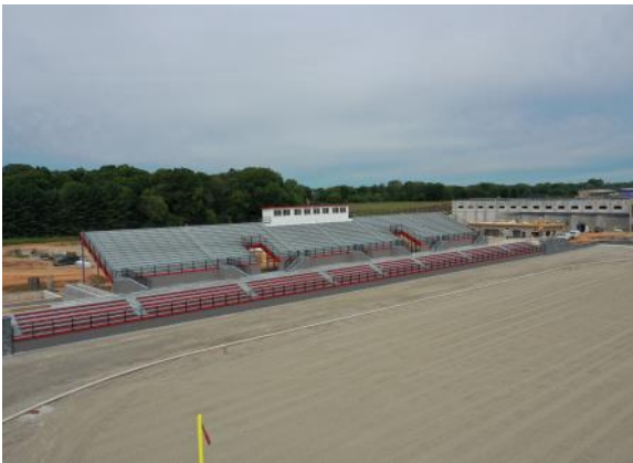
Aerial view of the grandstand bleachers (08/12/2022)
