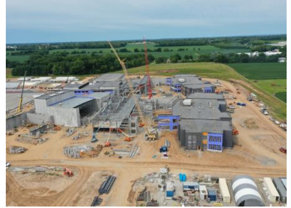
Aerial view of the building looking West (08/12/2022)
