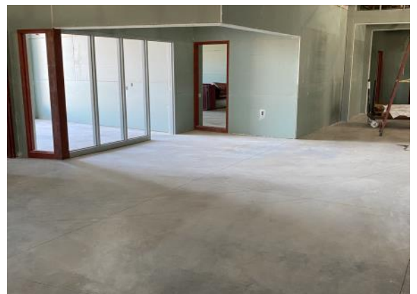
Drywall walls in academic classroom corridor (08/26/2022)
